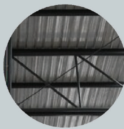
Metal pan roof with an open steel truss system
